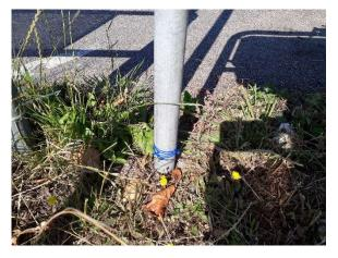
Close up you can see four blue bands of Cable tie/"plastic strip" so the code to write in the control card is "BBBB"
